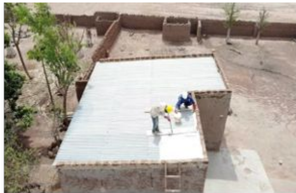
Application of cool roof coating
